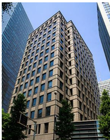
Mizuho Lease Building
