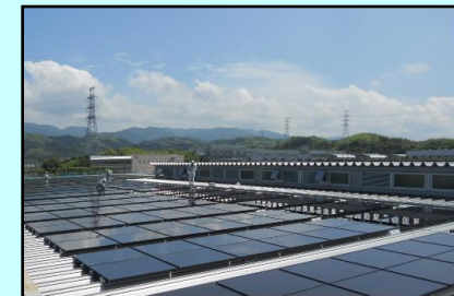
Solar power generation system
