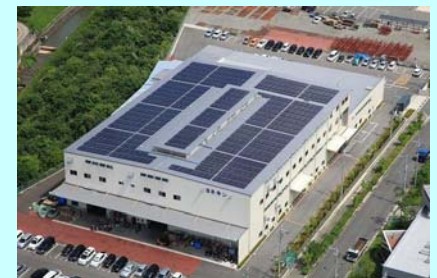
Solar power generation system on top of factory roof
