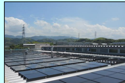
Photovoltaic device installed in customer plant
